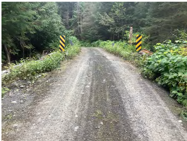
Approach from Left Bank when facing downstream
