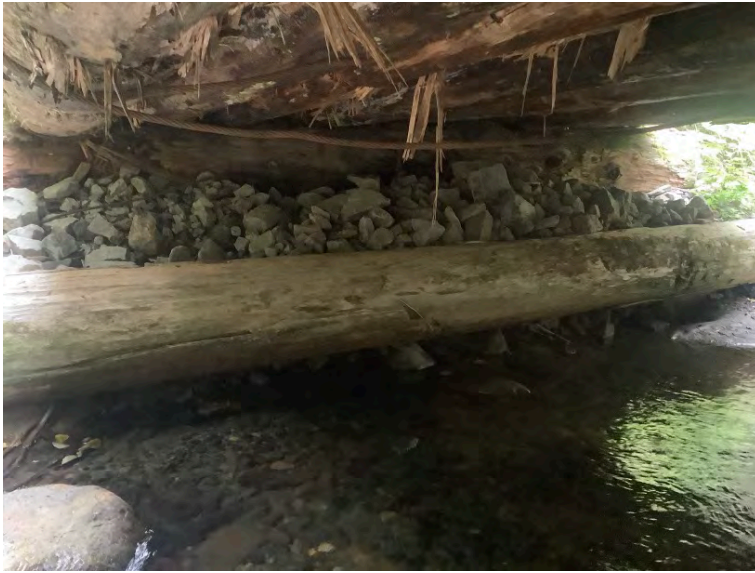
Right Bank Abutment when facing downstream
