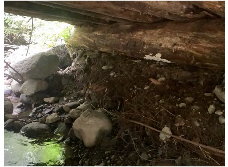
Left Bank Abutment when facing downstream
